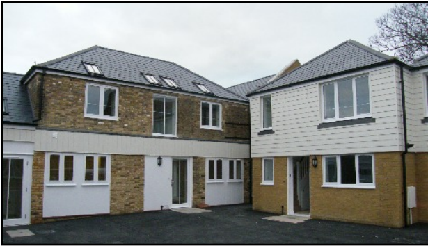
Above: Priory Mews, 8 The Square, Birchington - conversion of hay-store and new-build
