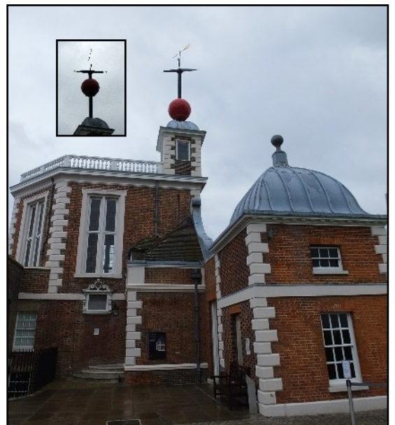
Flamsteed House with the Greenwich Observatory Time Ball with inset photograph showing position of the Time Ball immediately before it falls at 1.00pm each day
